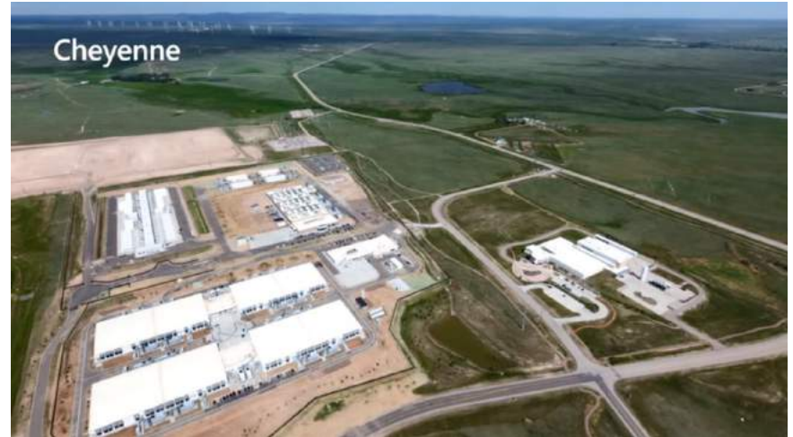
each facility is 8 MW in size, total of 64 MW
